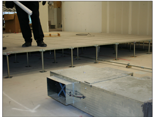
LHK terminal unit installed in an underfloor application
